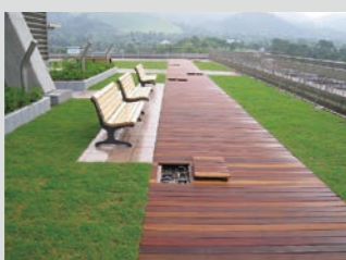
Super Soilen System Lightweight greening method
